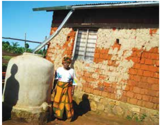
Rain water harvesting from roof top in Ibwera village, Kagera Region
