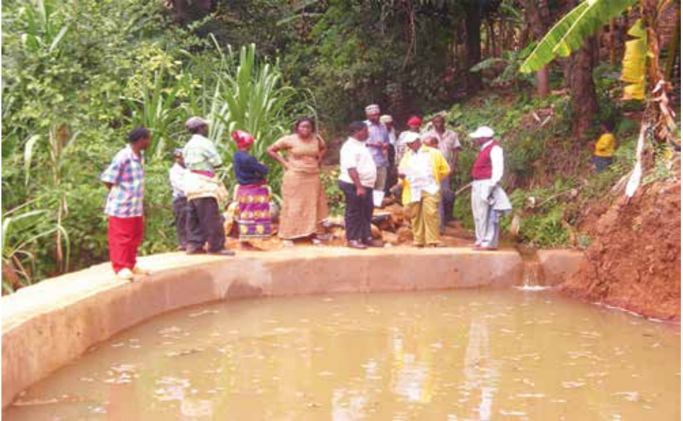
Stream flow diversion (Ndiva) at Mwembe village, Same district, Kilimanjaro
