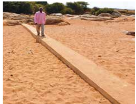
A subsurface water dam in Chololo village, Dodoma Municipality
