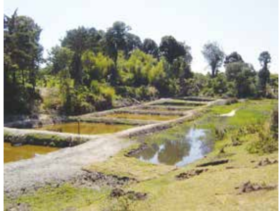
A series of earthen ponds at Mbinga, Ruvuma region which allows independent draining and filling.
